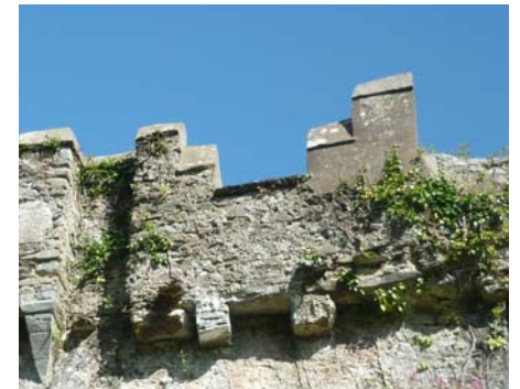
Detail view of drip stones & machicolations to south parapet
