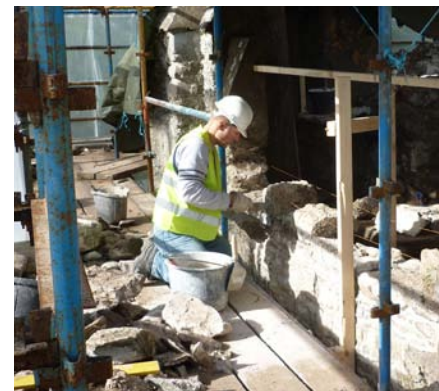
Parapet being rebuilt by Conservation & Restoration
