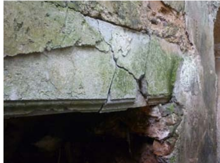
Detail of carved stone fireplace prior to repair
